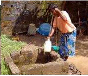
Unprotected Dug Well (C),
